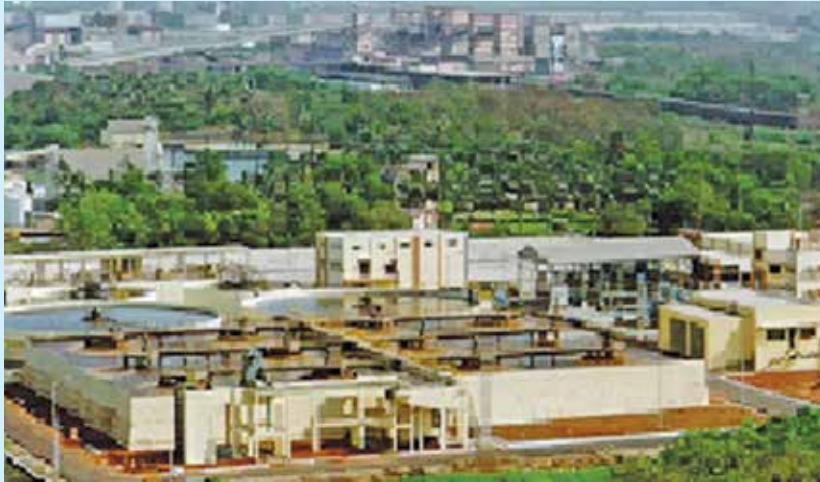
Bird eye view of Sewage Treatment plant.
