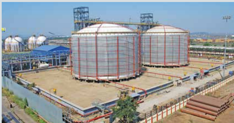
Bharat Petroleum's LPG Import Terminal at Uran
