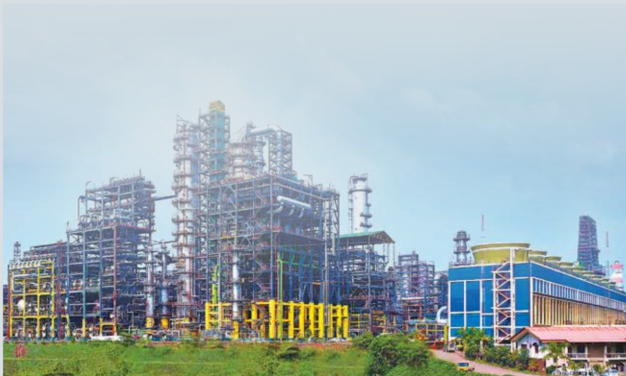
Bharat Petroleum's Integrated Refinery Expansion Project at Kochi.
