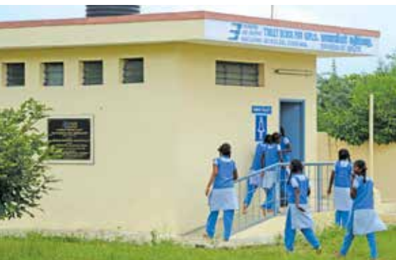
Toilets constructed for girls by CHN Unit under Swachh Vidyalaya Abhiyan.
