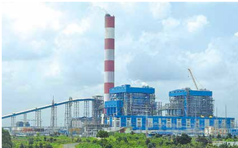
NTPC's Ultra Super Critical Plant at Khargone, M.P.
