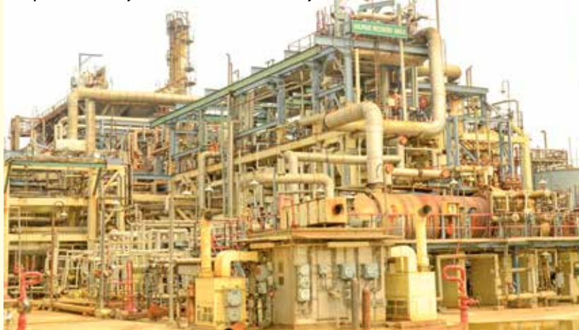
Sulphur recovery unit at Mathura Refinery.
