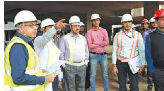
MD NHSRCL Mr. Achal Khare inspecting a High Speed Rail construction site at Vadodara, Gujarat.
