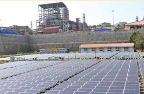
Solar project commissioned by MRPL.
