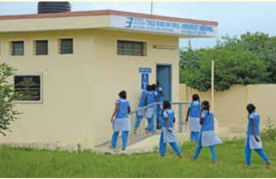
The toilet block constructed by BEL's Chennai Unit, under Swachh Vidyalaya Abhiyan, at Azhividaitangi village in Tamil Nadu. The village has been adopted by BEL.
