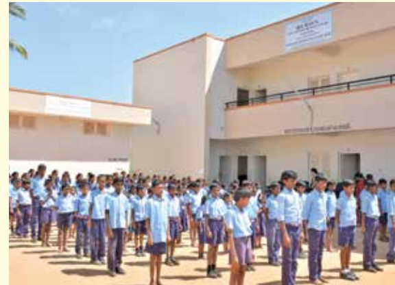
The new building and toilet block constructed by BEL at Government Higher Primary School, Kadaburu, Chikkaballapur district, Karnataka.
