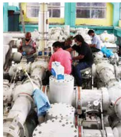
Gas Insulated Switchgear (GIS) restoration work under progress.
