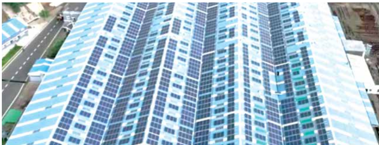
2 MWp project is one of the largest rooftop plant in Andhra Pradesh and on any government facility across India.
