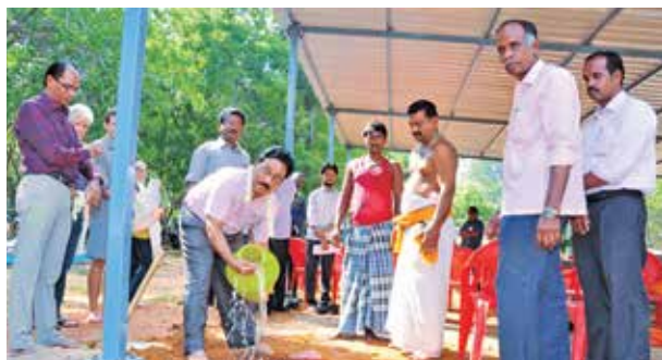
Bhoomi Puja for paver block road at Auroville, Pondicherry.
