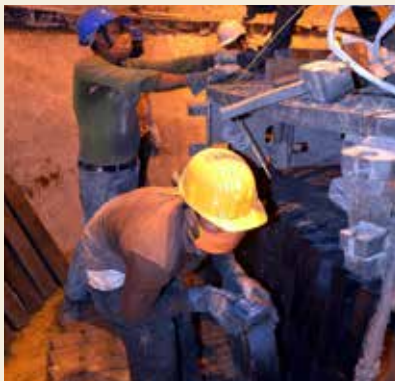
Refractory relining in Converter at SAIL-ISP going on.
