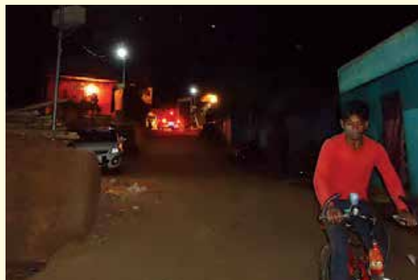
Solar Street Lights in a village, installed by NALCO.
