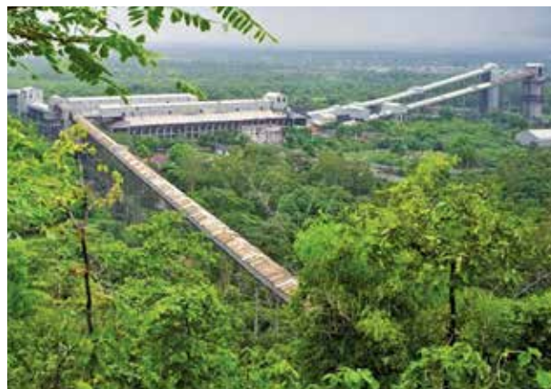
Green coal handling plant (CHP) at Nigahi project of NCL
