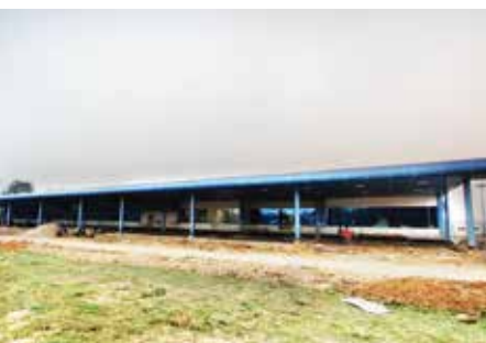
Work in Progress at Bokaro Airport.
