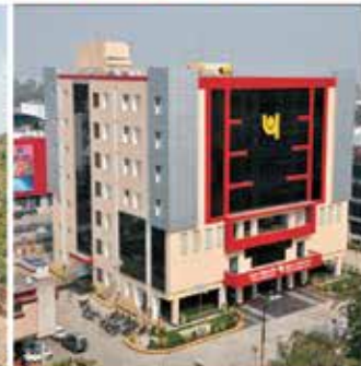
Punjab National Bank Regional Staff College Building at Lucknow
