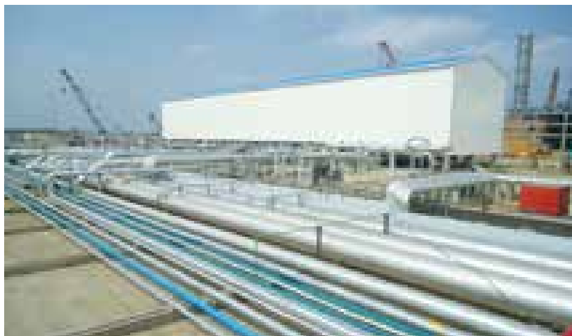
Crude Pump House IOCL Paradip Refinery, Odisha
