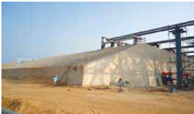
LPG Mounded Bullets Storage Facility IOCL Paradip Refinery, Odisha
