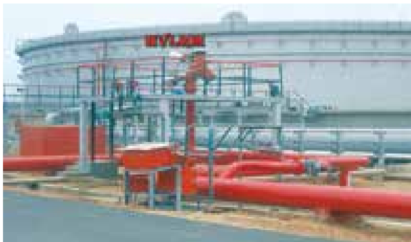
HVLRM – Fire Fighting Facility IOCL Paradip Refinery, Odisha
