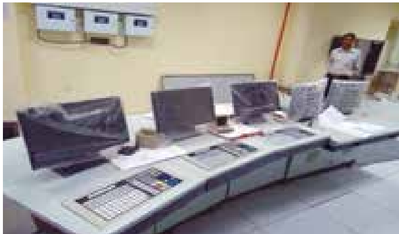
Crude Area Control Room IOCL Paradip Refinery, Odisha
