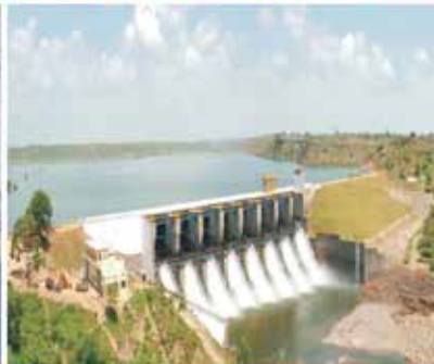
Shaheed Chandra Shekhar Jobat Dam, Jhabua M.P.
